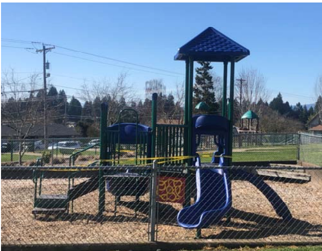
New play structure at Perkins Park
